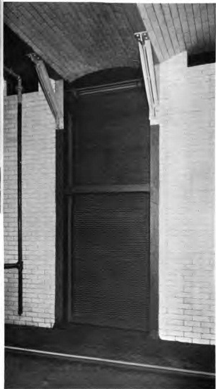
MANHOLES IN SIDE WALL OF SUBWAY
